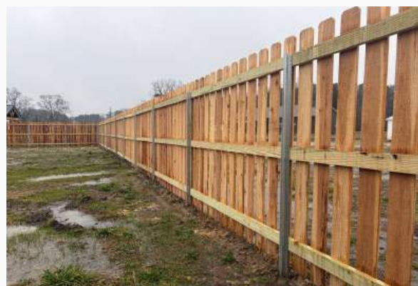
Steel Posts Upgrades
